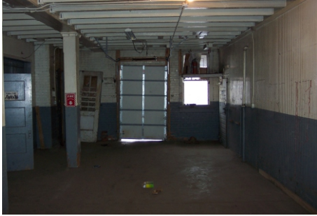
FIRST FLOOR BEFORE
