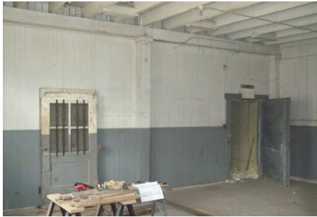
SECOND FLOOR: BEFORE
