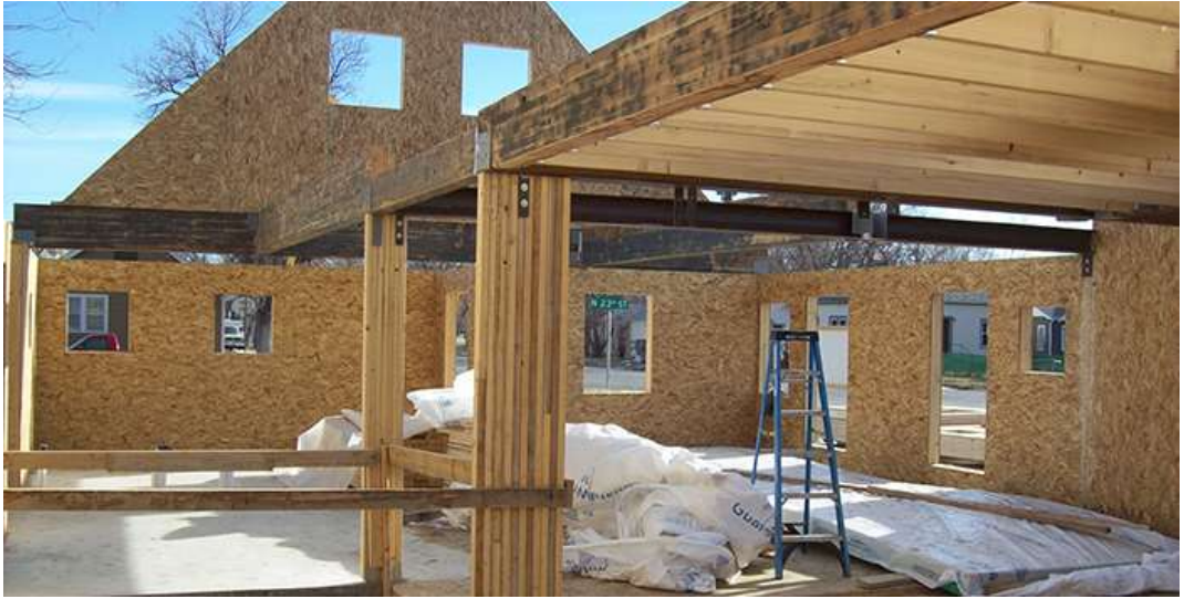
Starting the second floor floor
