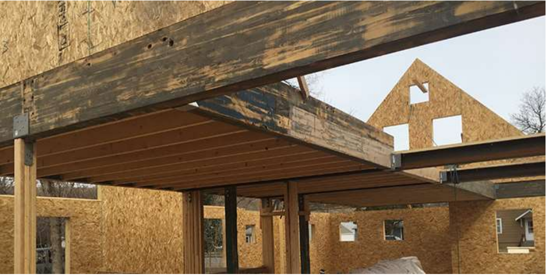
Beams from the old Lane Deer School
